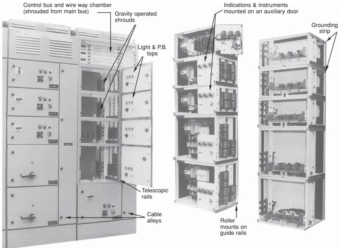
Figure 13.7(a) Details of a draw-out motor control centre (MCC) (Courtesy: ECS) (now Havells India)
