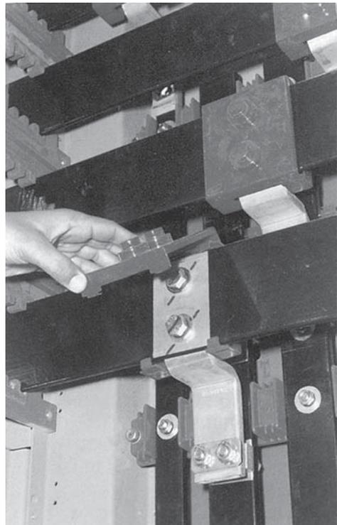
**Figure 13.37(b)** PVC/SMC/DMC/polycarbonate shrouds for bus joints and tap-offs
