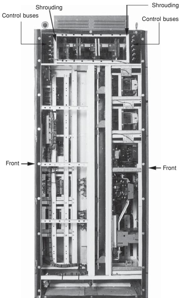
**Figure 13.4** Side view of a double front panel with a common horizontal bus, but separate vertical bus bars (not visible) (Courtesy: ECS) (now Havells India)
