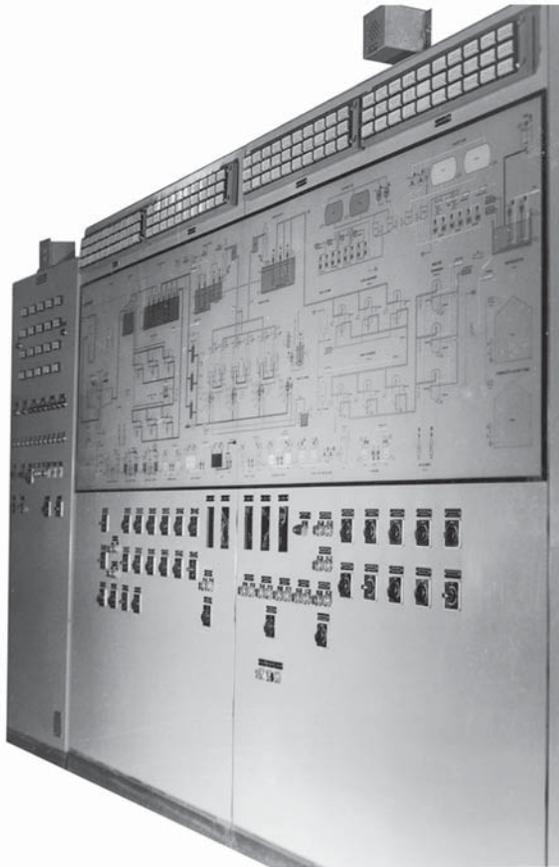
**Figure 13.10** A typical mimic-cum-process control panel (Courtesy: ECS) (now Havells India)
