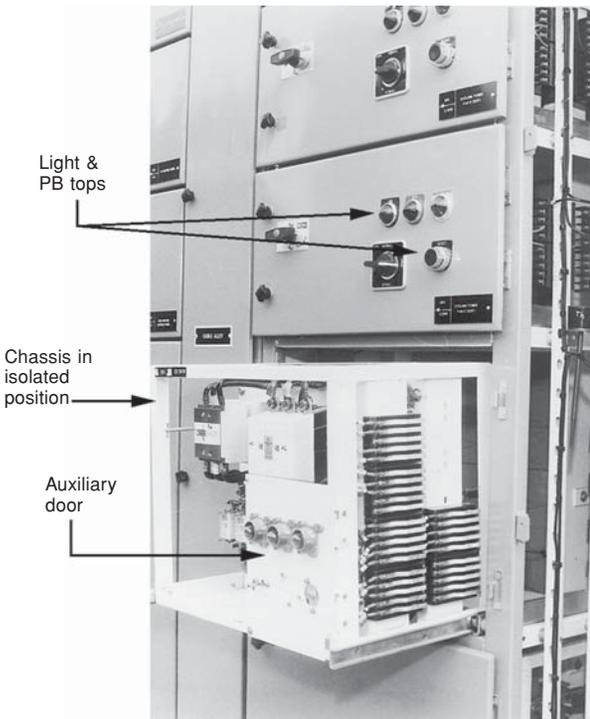
**Figure 13.8(a)** Part view of a typical fully draw-out type motor control centre (Courtesy: ECS) (now Havells India)
