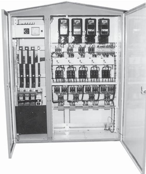
**Figure 13.2** A non-compartmentalized distribution board
