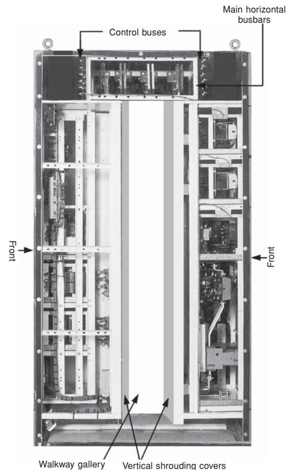
**Figure 13.5** A typical general arrangement of a double front panel with a walkway gallery
