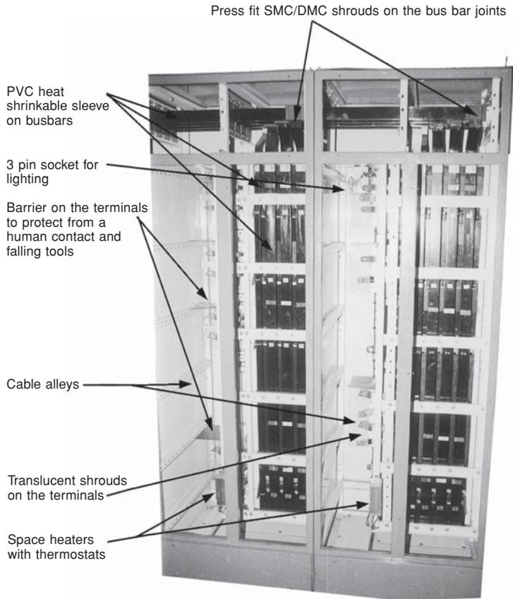
**Figure 13.34** Rear view of a typical MCC showing space heaters at the bottom of each cable alley and shrouding of the live parts (Courtesy: ECS) (now Havells India)
