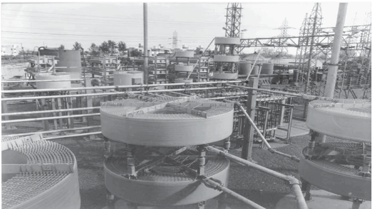
Figure 6.22(p3) SVC substation with shunt reactors in the foreground (Courtesy: Alstom)
