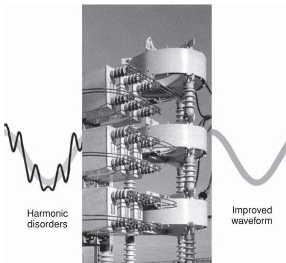
**Figure 27.14** A typical three phase tuning or filter reactor (Courtesy: ABB)
