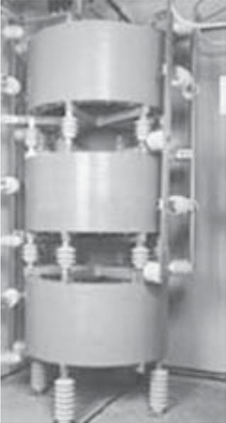
Figure 27.9(a) A typical 3-phase current limiting reactor (Source: Nokian Capacitors)
